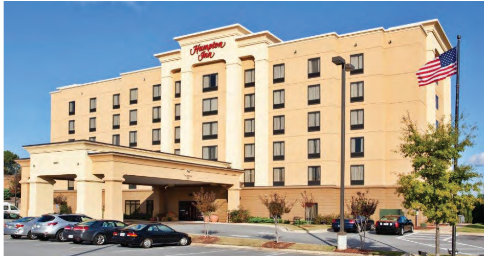
Royal Hotel Investments owns and operates this Hampton Inn in Covington, Georgia.
